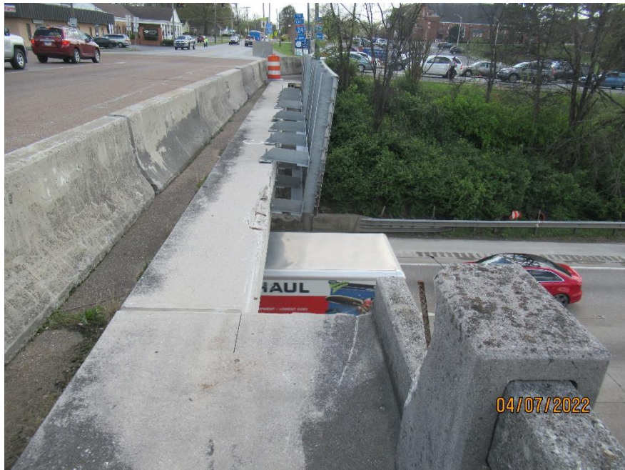
BEAM "A" REMOVED - SPAN #2 - LOOKING AHEAD
