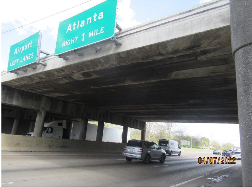
BOTTOM OF SPAN #2 - LOOKING AHEAD ON UNDERPASS
