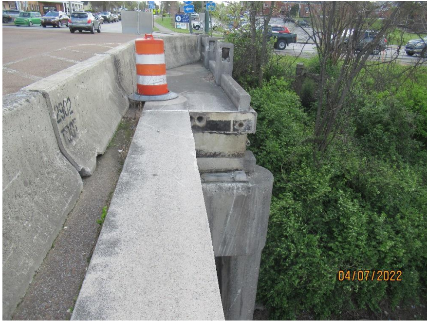
BEAM "A" REMOVED - BENT #1
