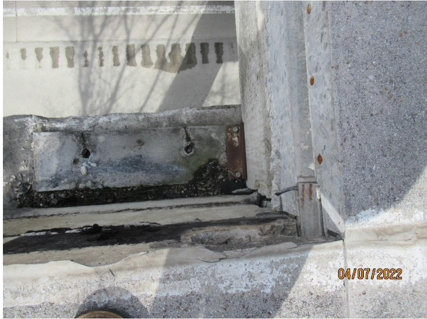
ANGLE IRON INSTALLED AFTER THE CURSORY INSPECTION OF 7-23-2020
