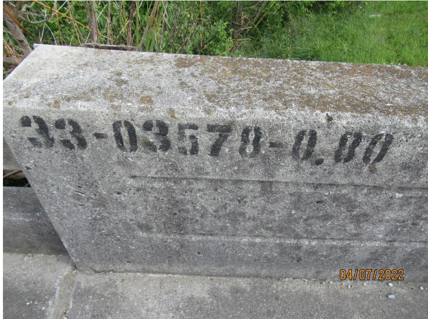
BRIDGE NO. - #1 RIGHT - BRIDGE RAIL
