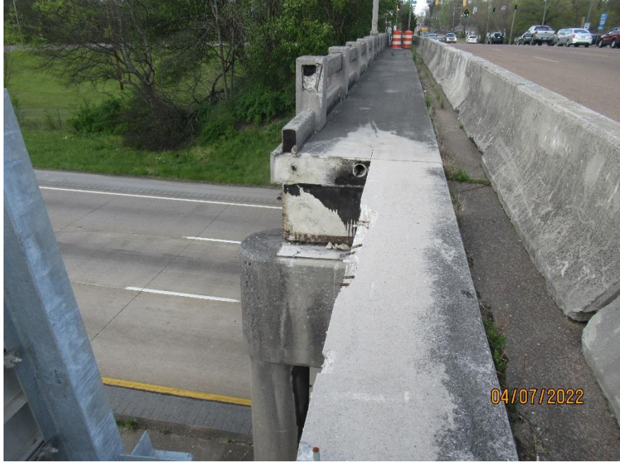
BEAM "A" REMOVED - BENT #2
