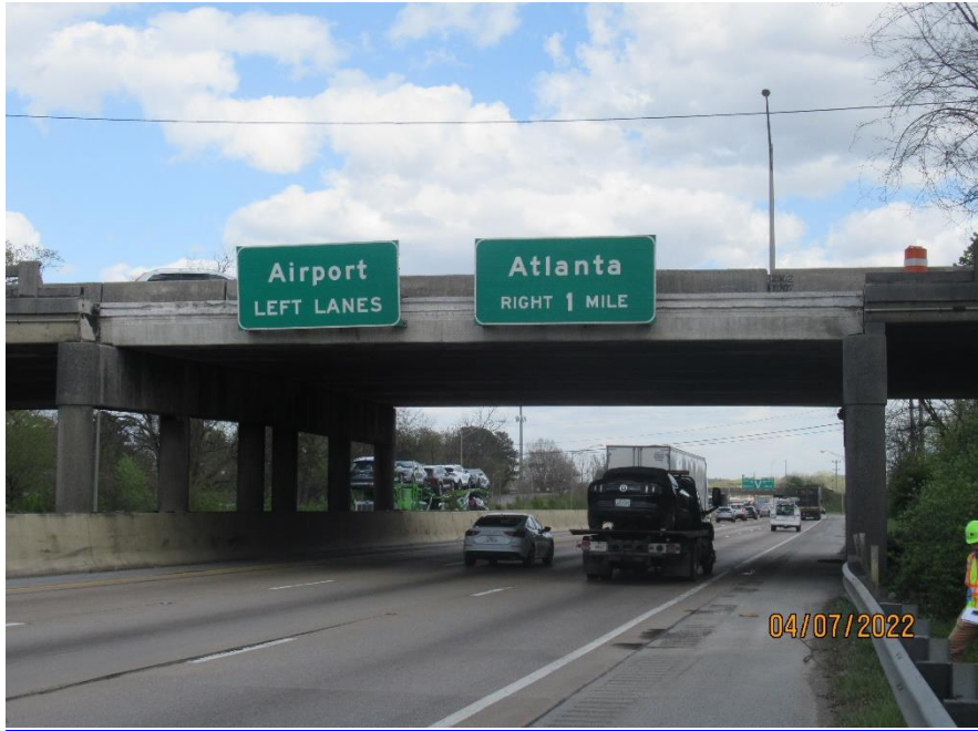
LEFT SIDEVIEW OF SPAN #2 - LOOKING AHEAD ON UNDERPASS
