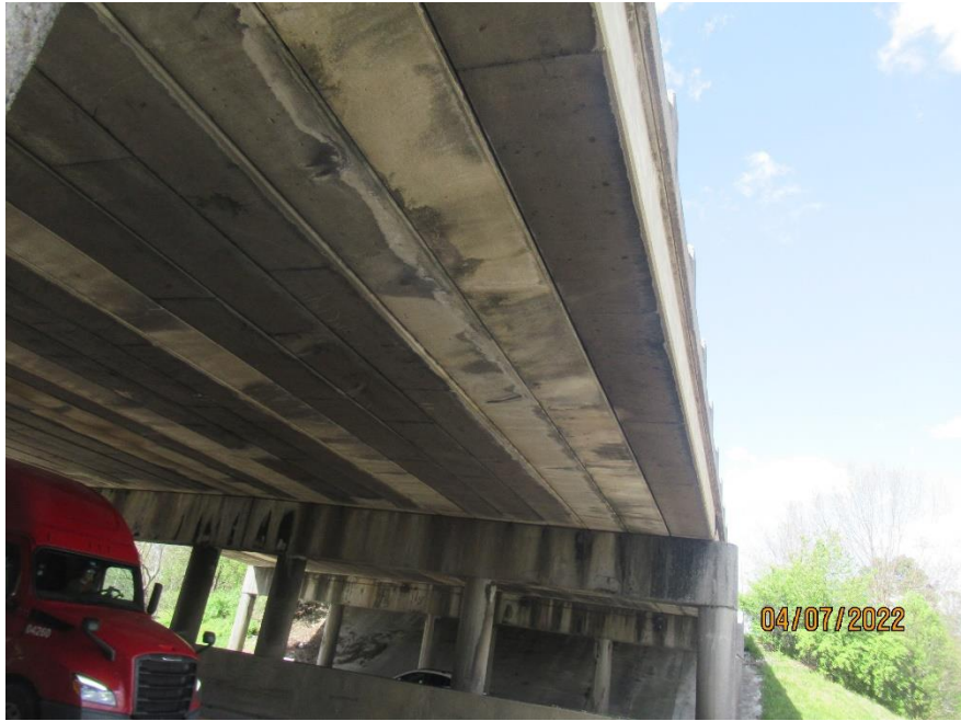
BOTTOM OF DECK - SPAN #2 - RIGHT
