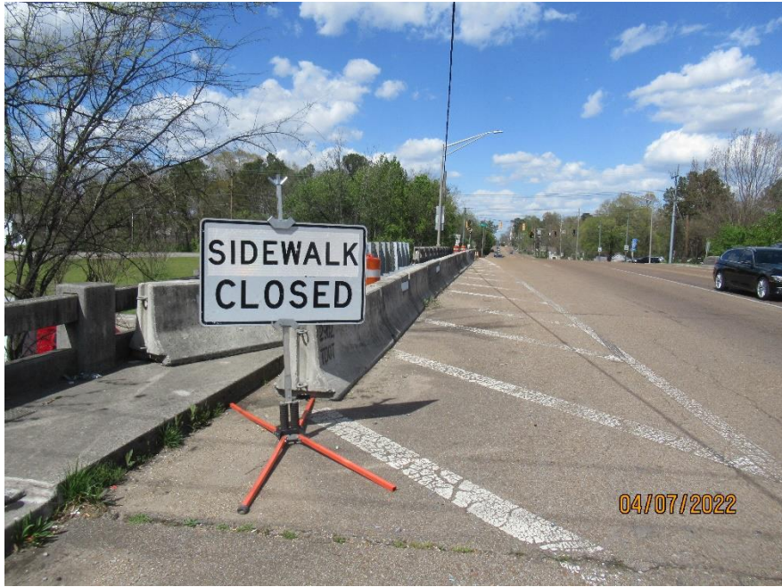
TRAFFIC CONTROL - LOOKING AHEAD
