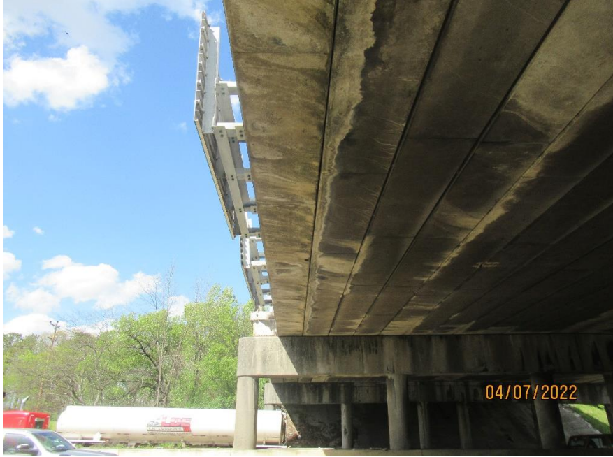
BOTTOM OF DECK - SPAN #2 - LEFT
